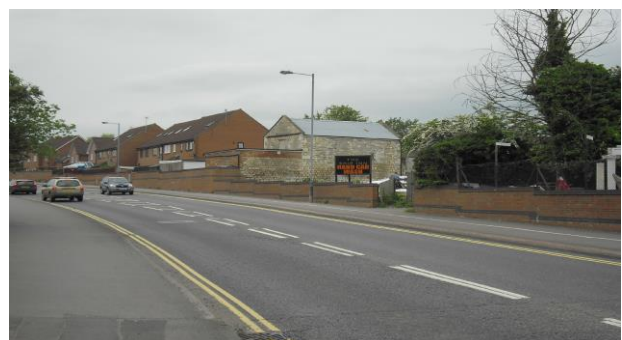
County Way/A361 public highway on site's southern boundary
